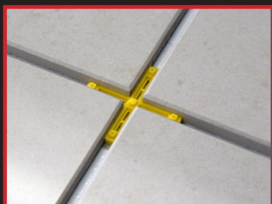
Leave-in grout joint & grout over
