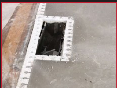
Easily trim flush after leveler is dry
