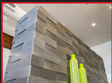
Lay wedge thick end-to-thin end
