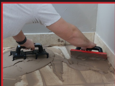
Ideal for troweling mortar on large format and GTP installations
