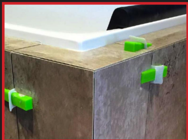
Keeps pieces from shifting or sagging while mortar cures
